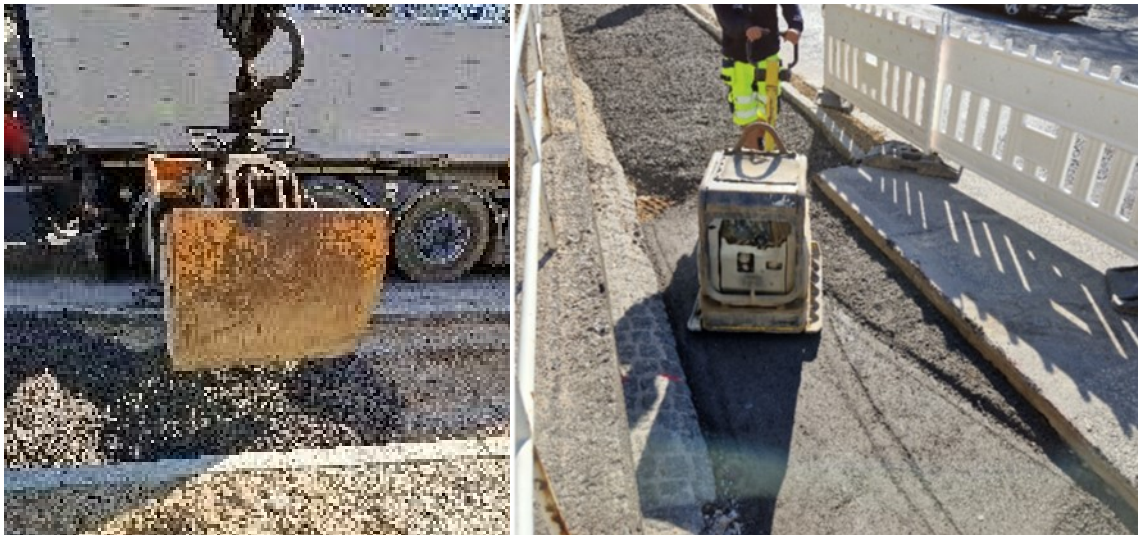
Bottom ash gravel used in a bike path.
