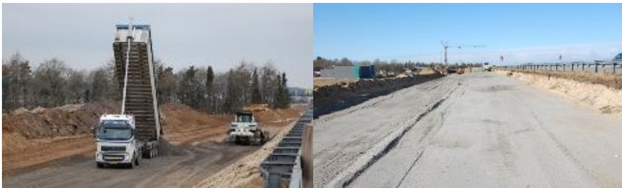
Example of bottom ash gravel used as subbase in roads.
